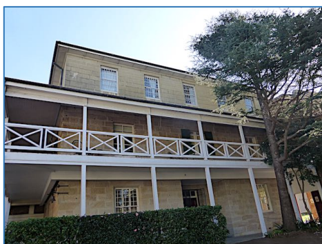
Section of original stone building of St Catherine's Waverley
